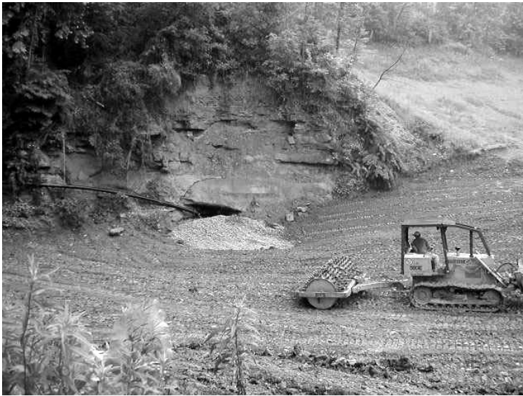
Perry Reclaiming workers filled the Congo Run subsidence hole with 155 tons of stone this June. Photo: Cara Hardesty.
